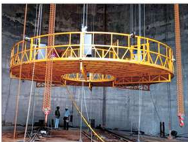
Chimney SRP, Mumbai
