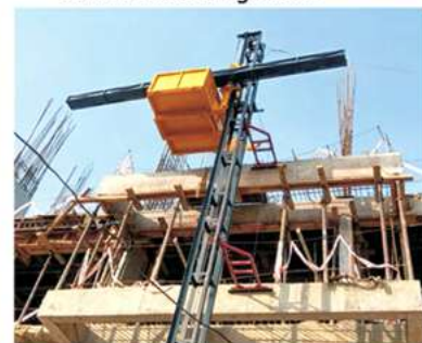
MFH - CMAC Rambo with Rebar Carrier, Delhi
